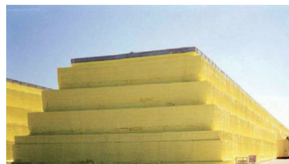
Figure 1. Example of megaton sulfur storage block nearly 18 m in height, courtesy of Alberta Sulfur Research Ltd.
